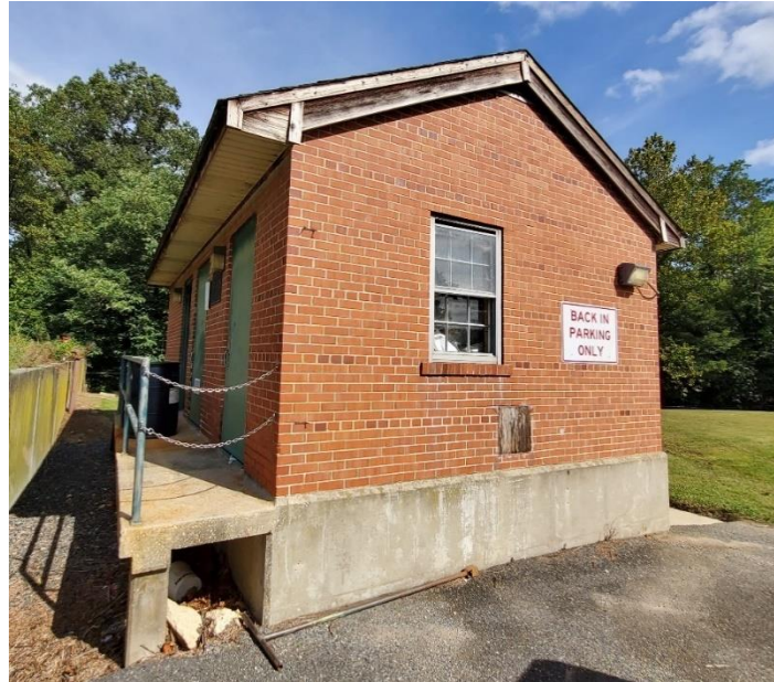
Figure 6.6: Existing Control Building
