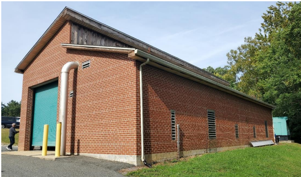
Figure 6.5: Existing Filter and Blower Building
