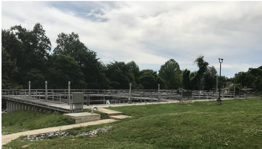
Figure 2.1: Centreville WWTP SBR
